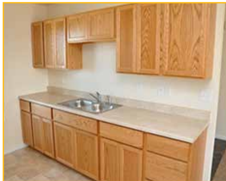
Sample Habitat for Humanity cabinets
